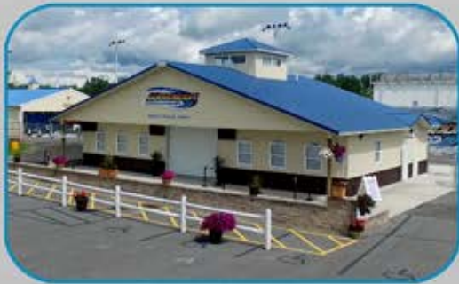
Entrance Building, Bathrooms, and Gearbox Retail Store
